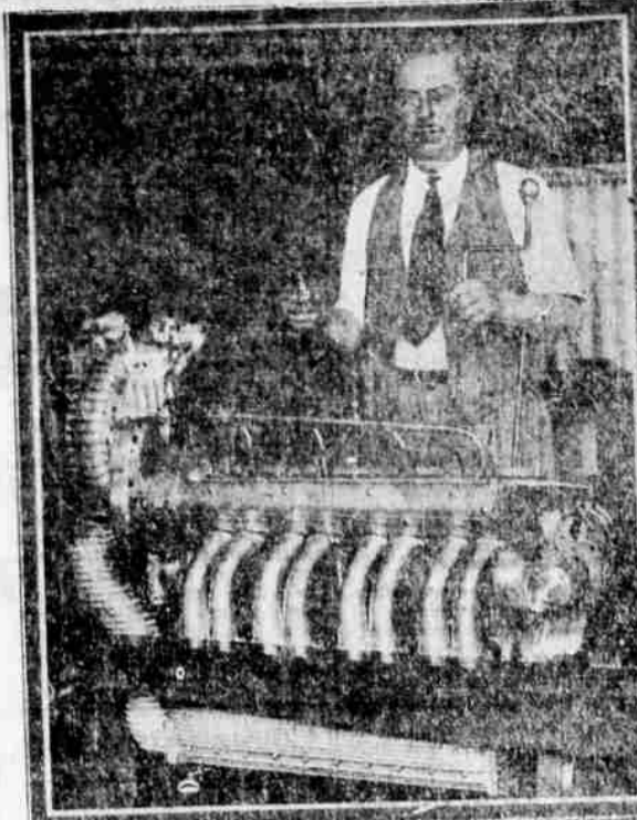
The tiny object in the hands of one of the world's most famous automotive engineers, Harry A. Miller, of Los Angeles, is a Champion spark plug he is going to place in one of the eight cylinders of a new 51-cubic-inch racing motor...
