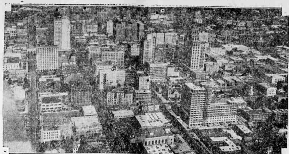
This is the latest skyline photo of Houston, Texas, where the Democratic national convention will be held in June. Below is an artist's drawing of the hall being erected to house the convention.
