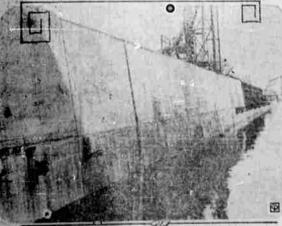
As spring approacher and with it the flood season, one river city, Beardstown, Ill., on the Illinois river, is counting on a new sea wall to protect it. The wall, pictured above, is 3,076 feet long and 22 feet high. It has just been completed. Earth levers, two miles long, connect the wall at each cod.
