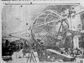
Work is well under way on the new glider boat, above, being constructed by the French engineer, Adrien Remy. He plans to use it in crossing the Atlantic between Cherbourg and New York, via the Azores. According to his calculations, the 17-ton craft can make the trip in 84 hours. The fusels is eiga haped and we contain the motor and cabins for passengers. Two floats, 79 feet long, will contain gasoline and oil tanks.
