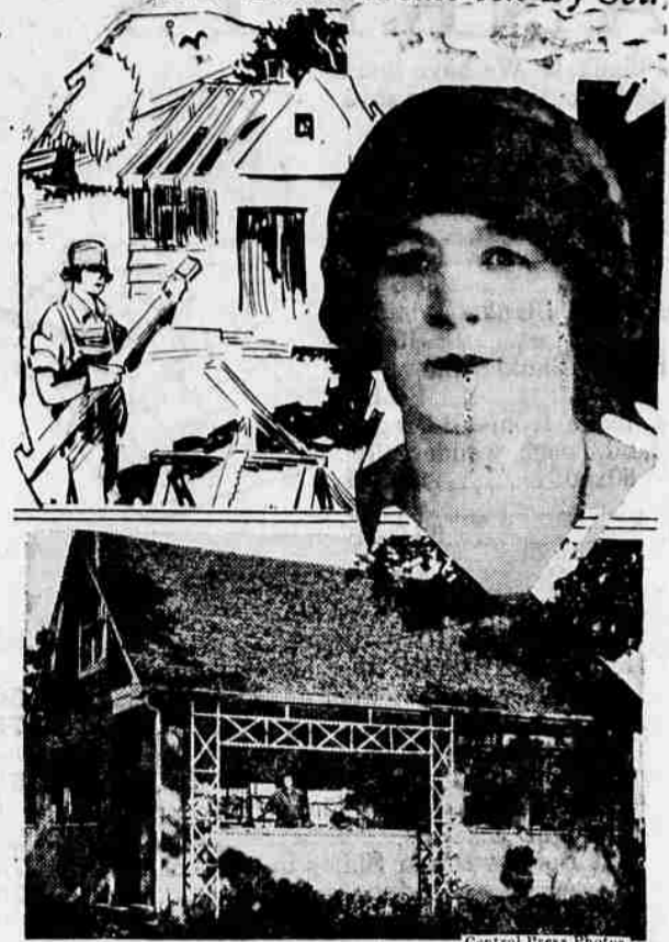
Want a house and short of funds? Build it all by yourself. Mrs. Lucile Lovely, Galesburg, Ill., proved that it can be done, even by a woman. She did all of the construction work on her new house, with the exception of a small amount of concrete-setting. House and Mrs. Lovely are shown.
