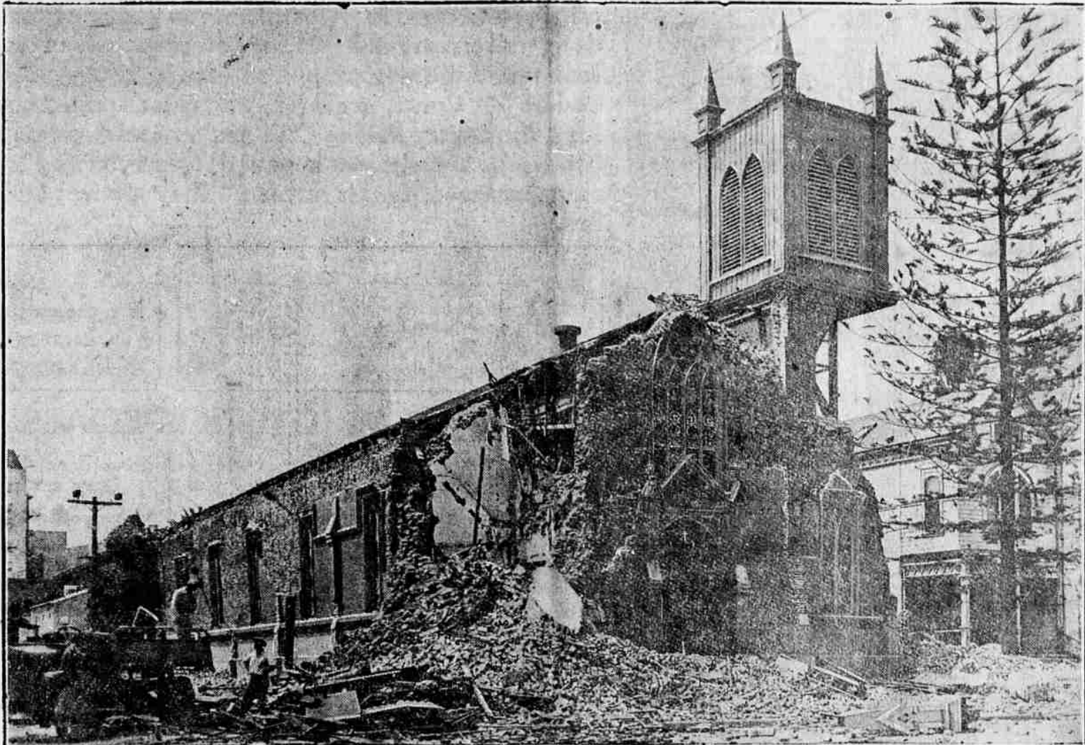
View at top shows all that remains of the Church of Our Lady of Sorrows on upper State street, near the Arlington Hotel. Below is a view looking up State street toward the Arlington Hotel from a point two blocks from the ocean.
