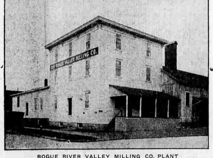
ROGUE RIVER VALLEY MILLING CO. PLANT
