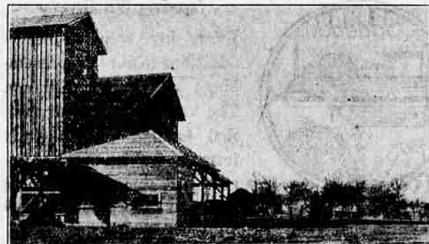
GENERAL VIEW OF PLANT AT CENTRAL POINT
