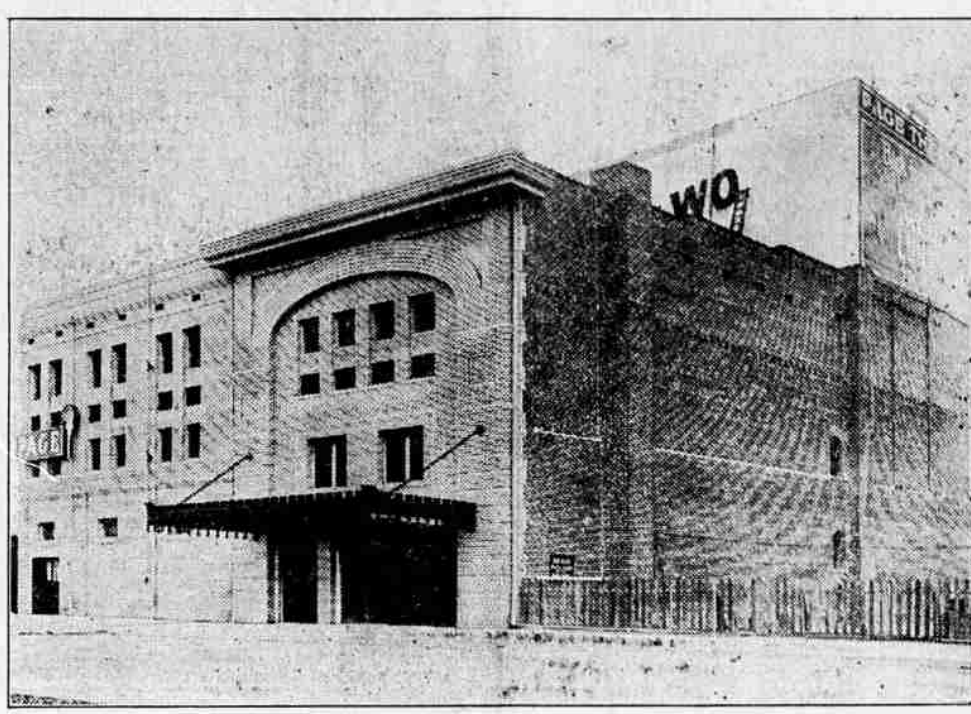
Above is shown the Page Theatre, the best and most modern playhouse in southern Oregon, which was completely gutted by fire early Sunday morning at a loss estimated at $100,000, partially covered by insurance. The origin of the fire is still a mystery, but it undoubtedly started in the northeast corner of the building, partly shown at the extreme left of the picture.
