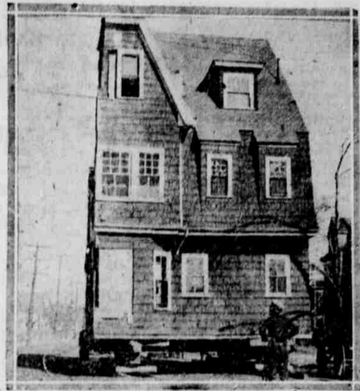
This half of a three-story house was photographed while being moved along Commonwealth Ave., Newton, Mass., the section weighing approximately 40 tons. It is being moved a distance of one quarter of a mile from its original spot.
