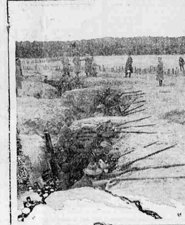
Digging trenches about suburbs of Berlin and training of civilians during the day of the world's reckoning.
