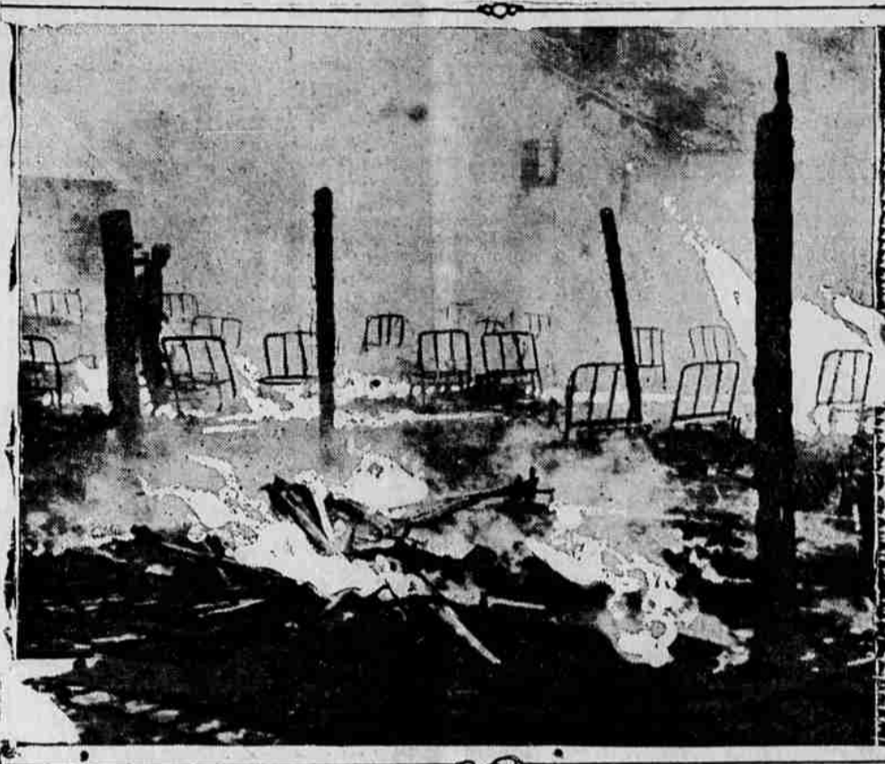
Here is photographic proof of the stories about Germans firing on hospitals and other buildings of the Red Cross. This French war hospital near the front was made the target for German shells, which demolished it thoroughly and set the ruins afire. Note the rows of iron beds, twisted and blackened by the flames.
