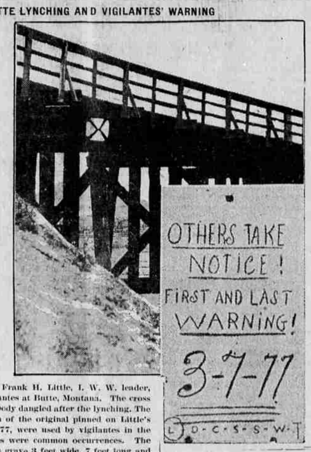
View of railway trestle from which Frank H. Little, I. W. W. leader, was hanged recently by a mob of vigilantes at Butte, Montana. The cross marks the girder from which Little's body dangled after the lynching. The warning shown above is a reproduction of the original pinned on Little's body by his captors. The figures, 3-7-77, were used by vigilantes in the days of the old west when lynching bees were common occurrences. The numerals designate the dimensions of a grave 3 feet wide, 7 feet long and 7 1/2 inches deep, the regulation measurements of a grave. The initials at the bottom of this gruesome tag are supposed to represent the names of other men who have been active in I. W. W. work with Little. To the left is Frank H. Little.
