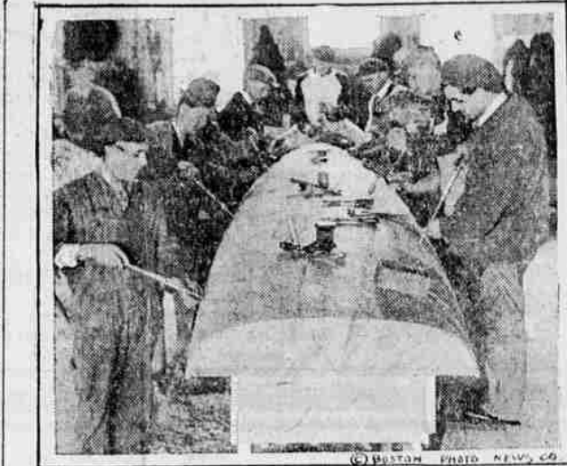
Fastening mahogany bottoms to the pontoons of seaplanes being constructed for Uncle Sam. Twenty-two thousand six hundred and twenty-five aircraft are planned and engines for them will cost approximately $363,000,000 and the remaining $276,000,000 asked would be necessary to man the air fleets and provide for ammunition and supplies.
