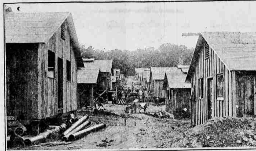
The cantonment city of the U. S. marine corps at Quantico, Virginia—a type of the 16 others now being rushed to completion. Above is shown a row of houses on the freshly cleared land with the primeval forest in the background; below is a typical street between the almost finished dwellings where men selected for service will live while being trained.
