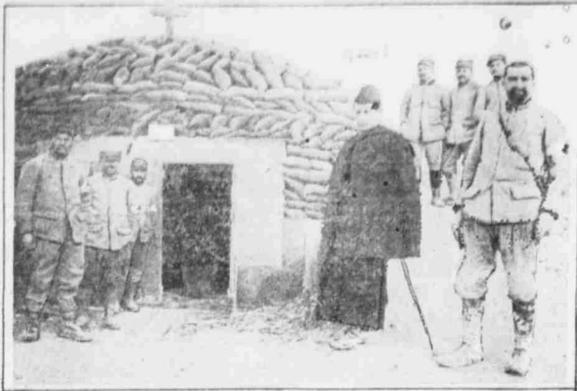
A unique church "somewhere" in the Champagne region in France which is built practically on the firing line. The auditorium of the church is underground while nine layers of sand bags cover it to protect it from bursting shells. The clergyman is shown to the right of the entrance.
