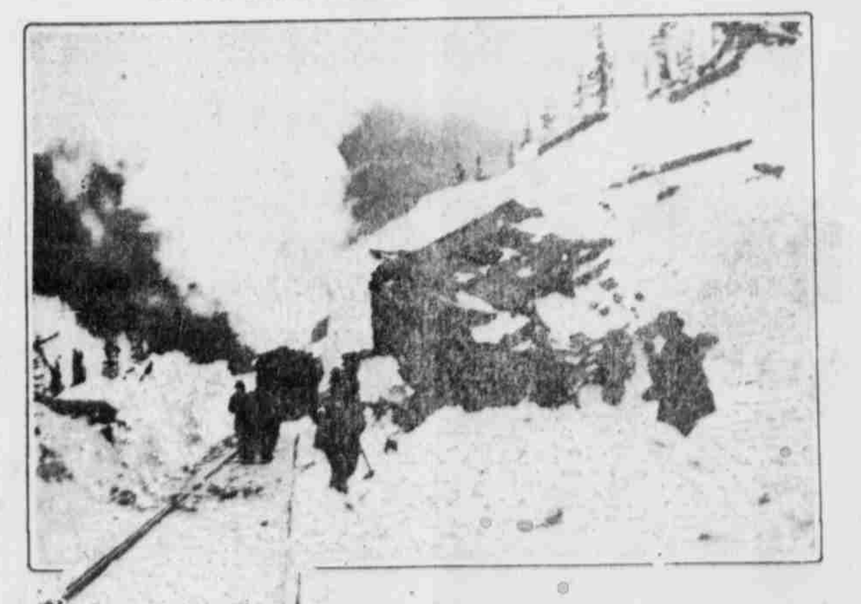
Wrecked day coach of the Great Northern train, lying at the edge of the lower track after being carried down the 400-foot slope by an avalanche of snow recently near Corea station, Washington. It was in this coach that nearly all of the eight persons who died met their doom. A rotary snow plow has just cleared the lower track for the rescue party.
