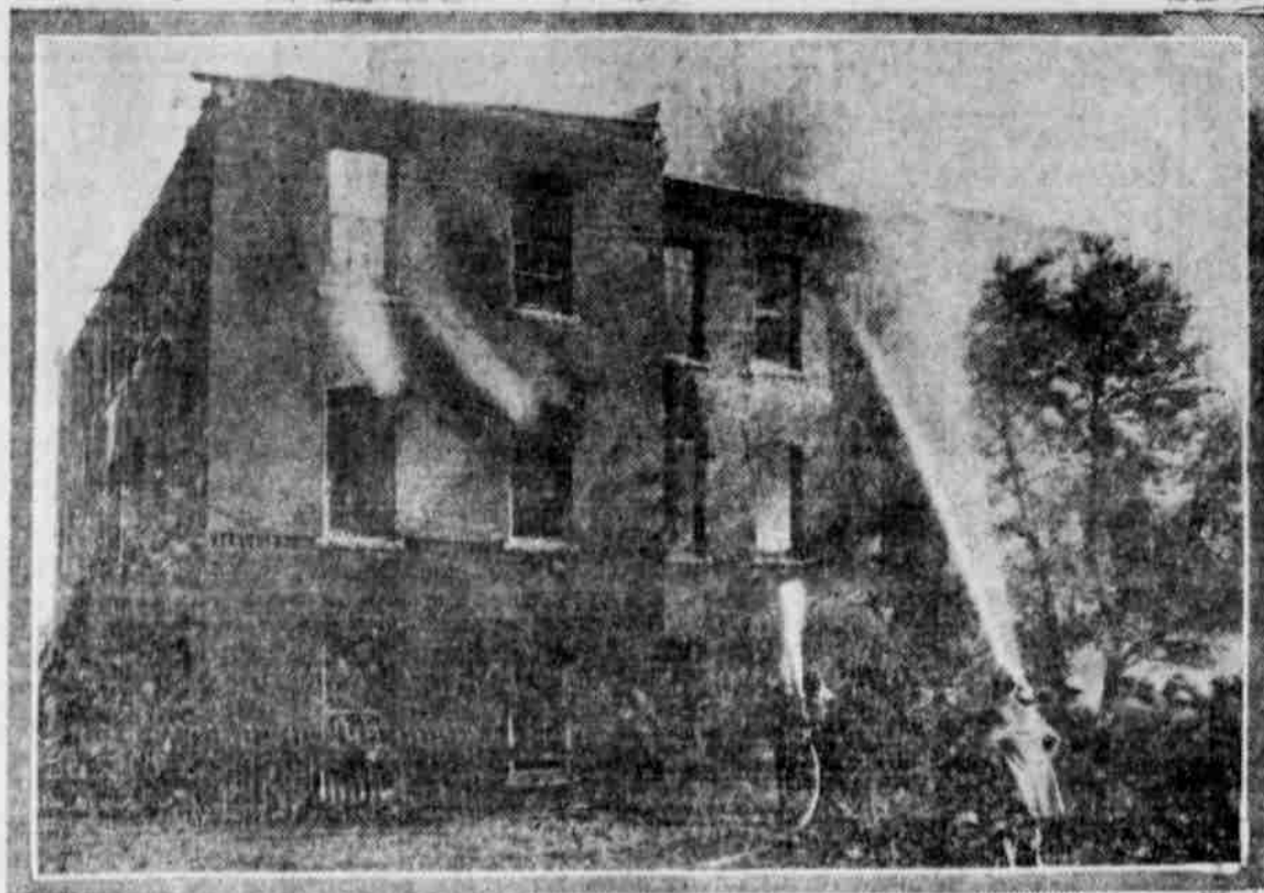
This is St. John's Parochial school at Peabody, Mass., where twenty-two young girls were burned to death in a fire that destroyed the inside of the building Thursday. Note that the three-story structure has no fire escapes. Many of the lives were lost when the little victims jumped from the windows; others were smothered or crushed under their comrades' heels before they could reach safety.
