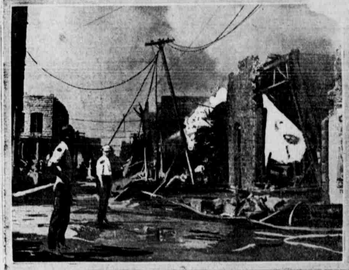
This picture shows a scene in the business district of Ardmore, Okla., after the explosion of a tank of gasoline on a Santa Fe railroad car which killed forty and injured several.
