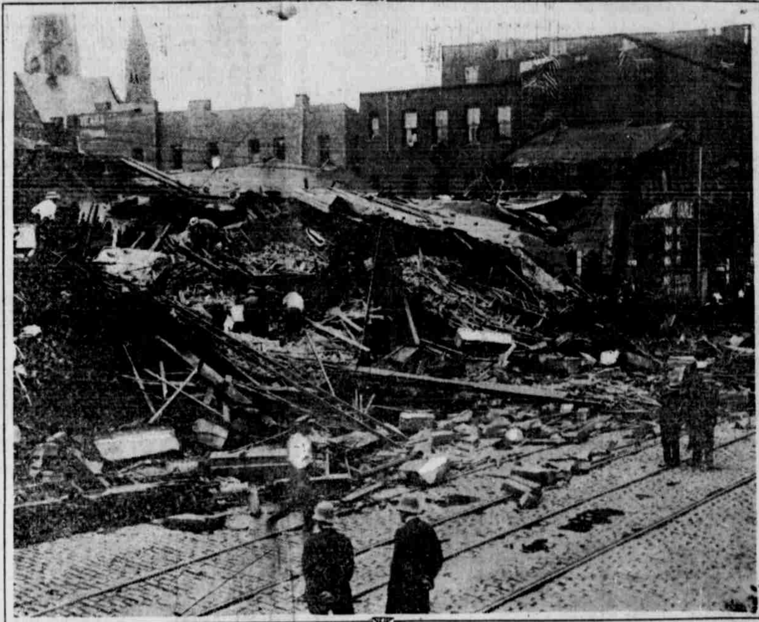
After the cyclone had passed over West Sixth Street, Cincinnati, photograph shows men searching the wreckage of what had been houses for buried victims.
