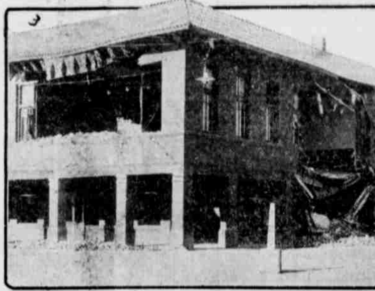
Masonic Temple, El Centro, wrecked by quake.
