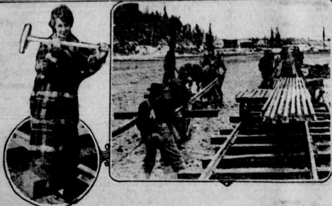
Views in the new land of opportunity—at left, Miss "Babe" White driving first spike for $31,000,000 government railroad in Alaska; above, a "sour-dough" camp at Strip Creek, now Anchorage; below, laying the terminal track at Anchorage beach.
