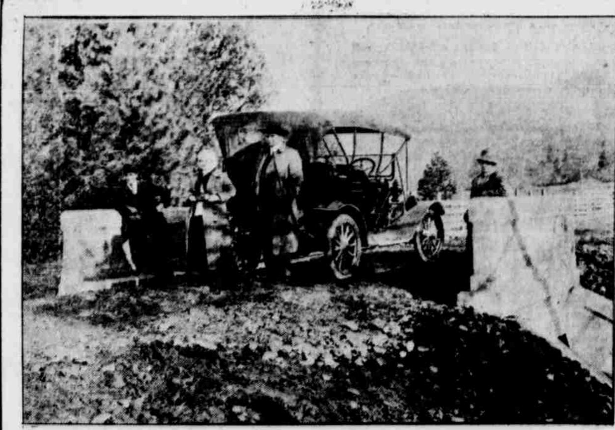
CULVERT, ON POSTAL HIGHWAY
