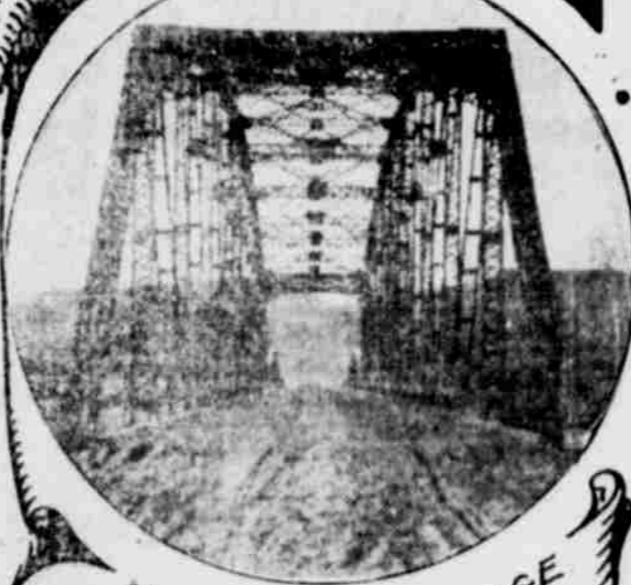
NEW MODOC BRIDGE OVER ROGUE RIVER
