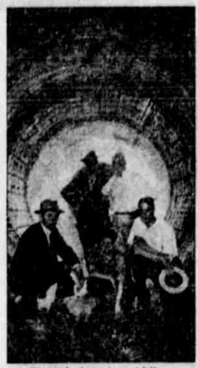
Scene in interior of kiln.
