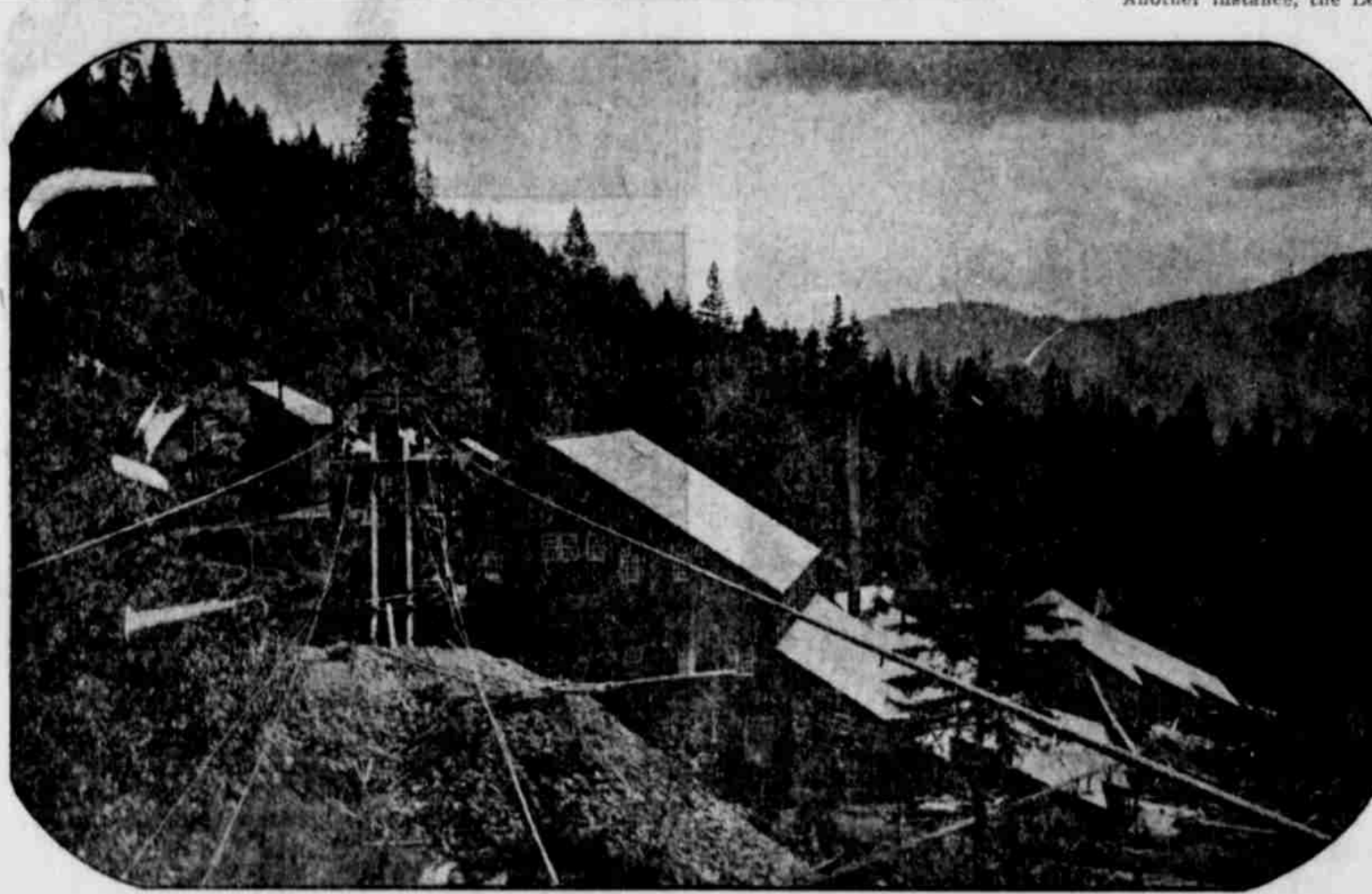
Quartz Mill at the Greenback, One of the Few Mines Which Have Been Dug to Any Depth Below the Grass Roots.
