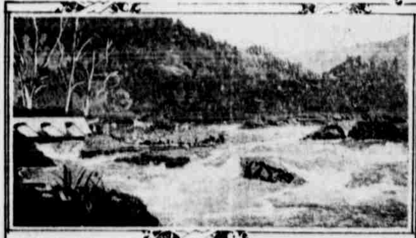
Power Plant at Gold Hill Now Nearing Completion.
