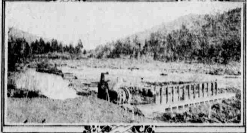
Top, Lower Portion of Twenty-Foot Fall—Middle, Control Gates—Below, Head Gates Waiting For Water
