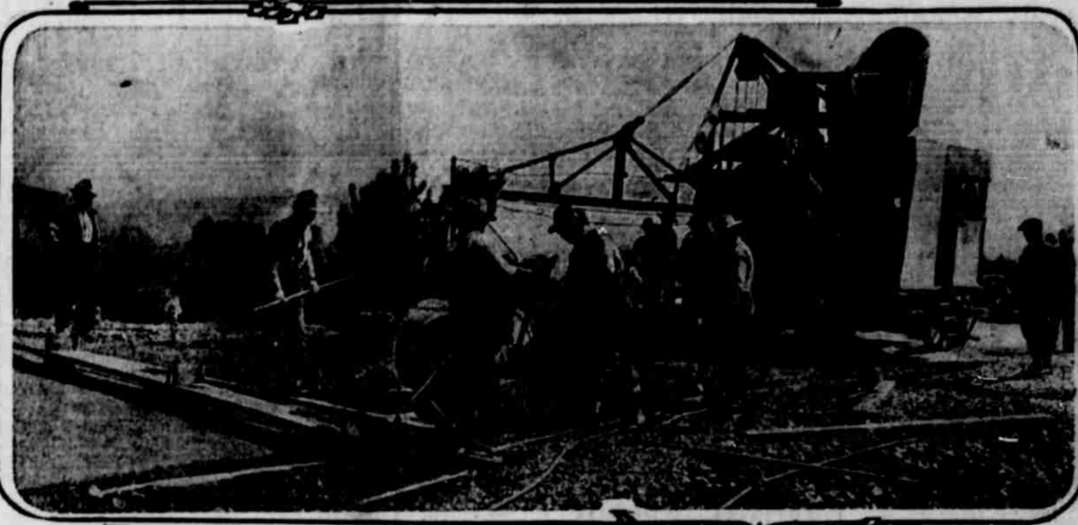
SCENES SHOWING LAYING OF GRANITOID-CEMENT PAVING ON PACIFIC HIGHWAY
