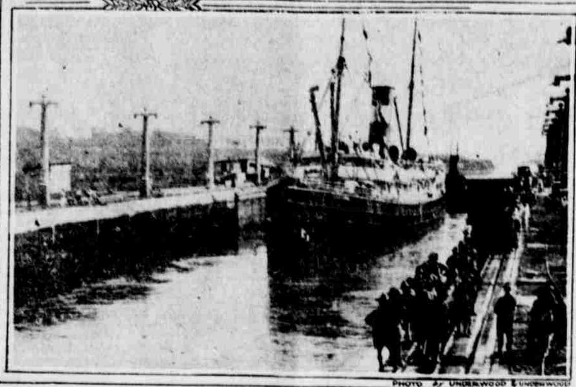
The steamship Alliance, belonging to the Panama Railroad Company, is the first large vessel to pass through the Gatun locks of the Panama Canal. It was on June 8 that she was sent through the locks for the purpose of testing the electric locomotives that will be used to tow vessels through the locks. The test was a success, the locomotives handling the four thousand ton steamship easily and speedily. It took the Alliance one and one-half hours to pass through the locks.
