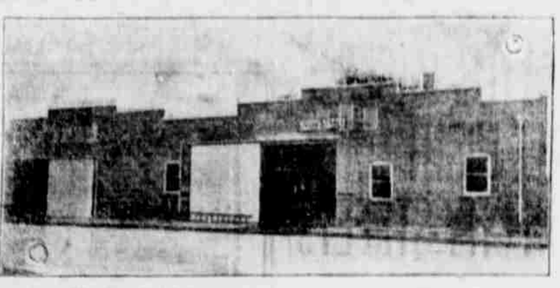
The New Brick Union Livery Barn on South Riverside Everything new and up-to-date. Livery and ambulance service.
