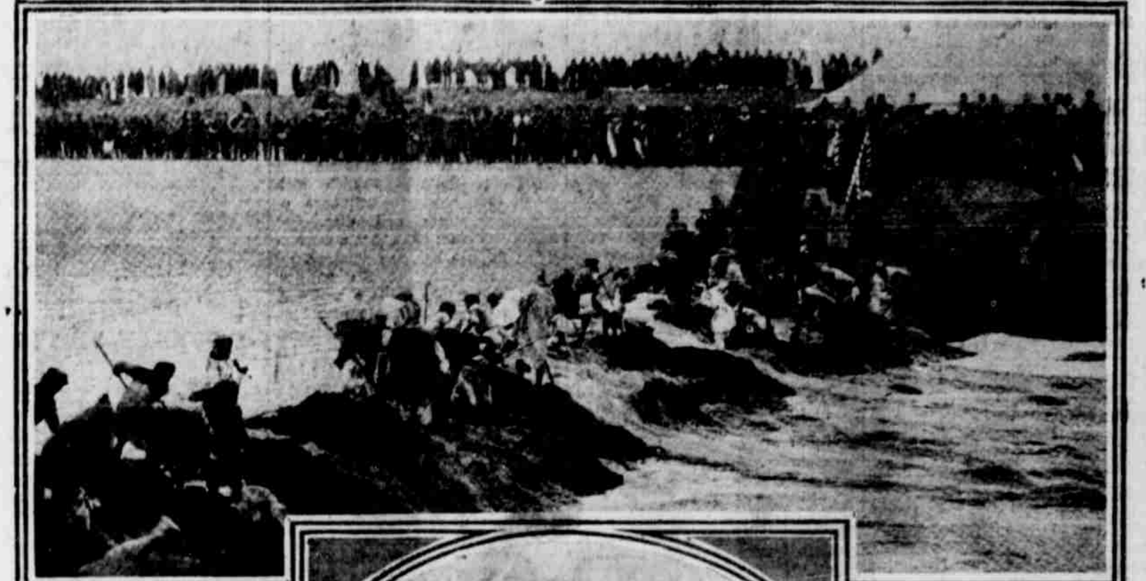
THE FIRST WATER IN THE HILLA CANAL
