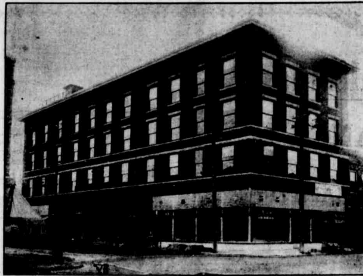
Garnett-Corey Hardware Company Building
