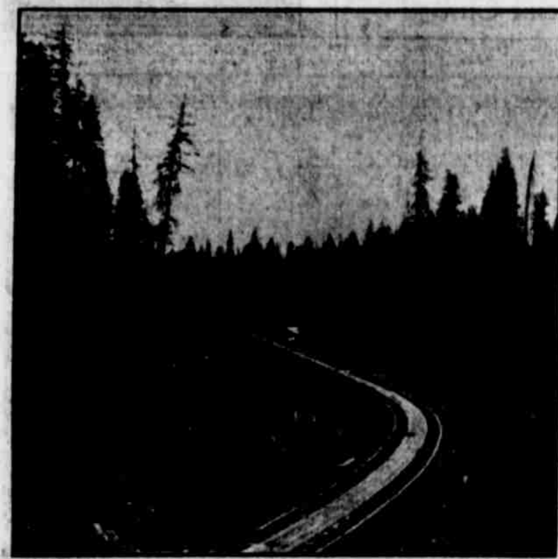
Flume Carrying Water to Drop
