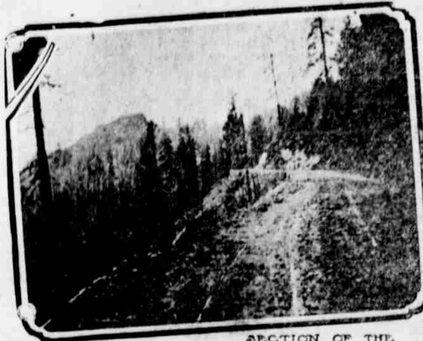
Construction Scenes in Jackson County Road Building.
