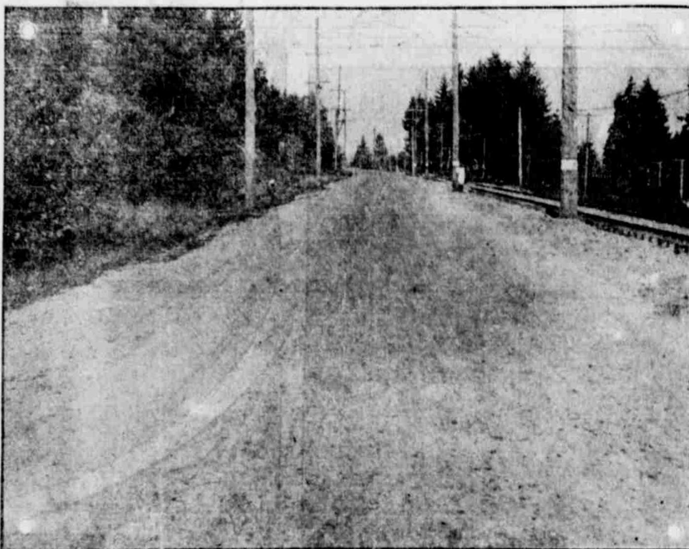
The First Hard-Surface Road Laid in Oregon THE LINNTON ROAD, MULTNOMAH COUNTY Paved With WARRENITE
