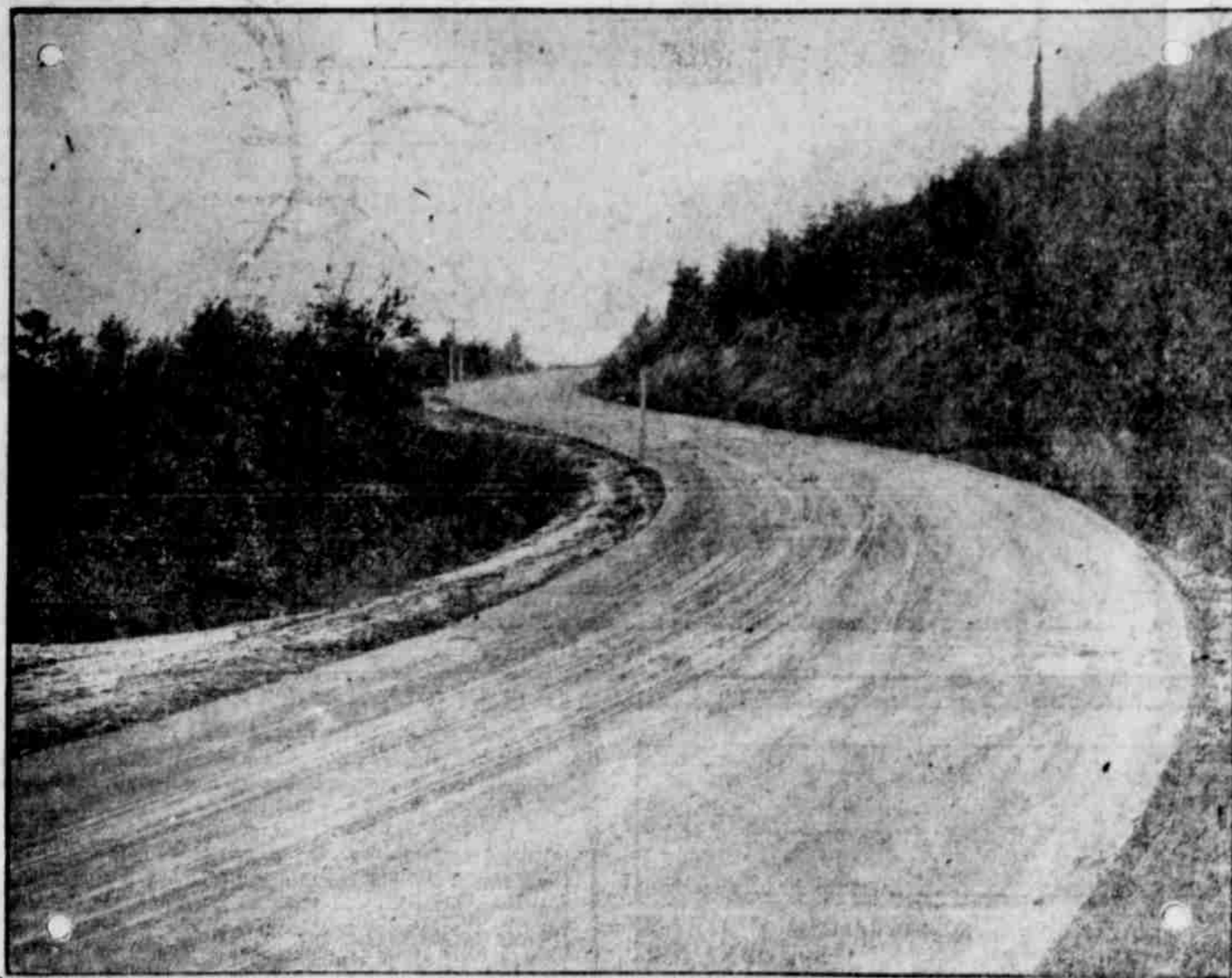
The TERWILLIGER BOULEVARD, Portland, Oregon Paved With WARRENITE
