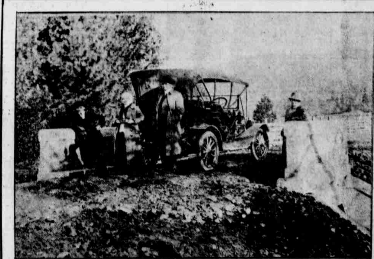
CULVERT ON POSTAL HIGHWAY
