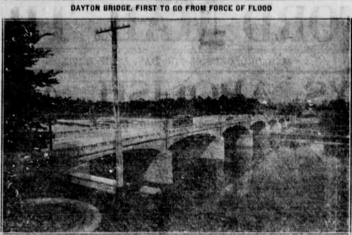
DAYTON BRIDGE, FIRST TO GO FROM FORCE OF FLOOD. This substantial concrete structure withstood the force of the Ohio flood for a very short time. It was one of the principal thoroughfares of Dayton, but when the water rose to the river banks the force was so great that the bridge was carried out.
