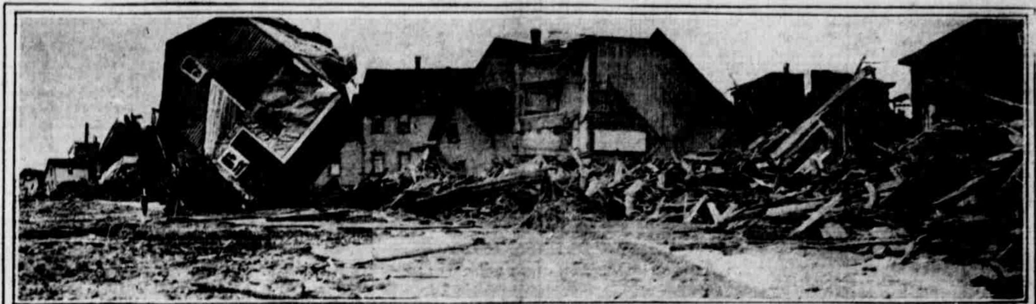
RUINS IN OUTSKIRTS OF OMAHA. In this picture is shown an actual scene in Omaha, Neb., following the great cyclone which caused so much damage and loss of life. The destruction shown here is only a small part of the devastation caused by the awful storm.
