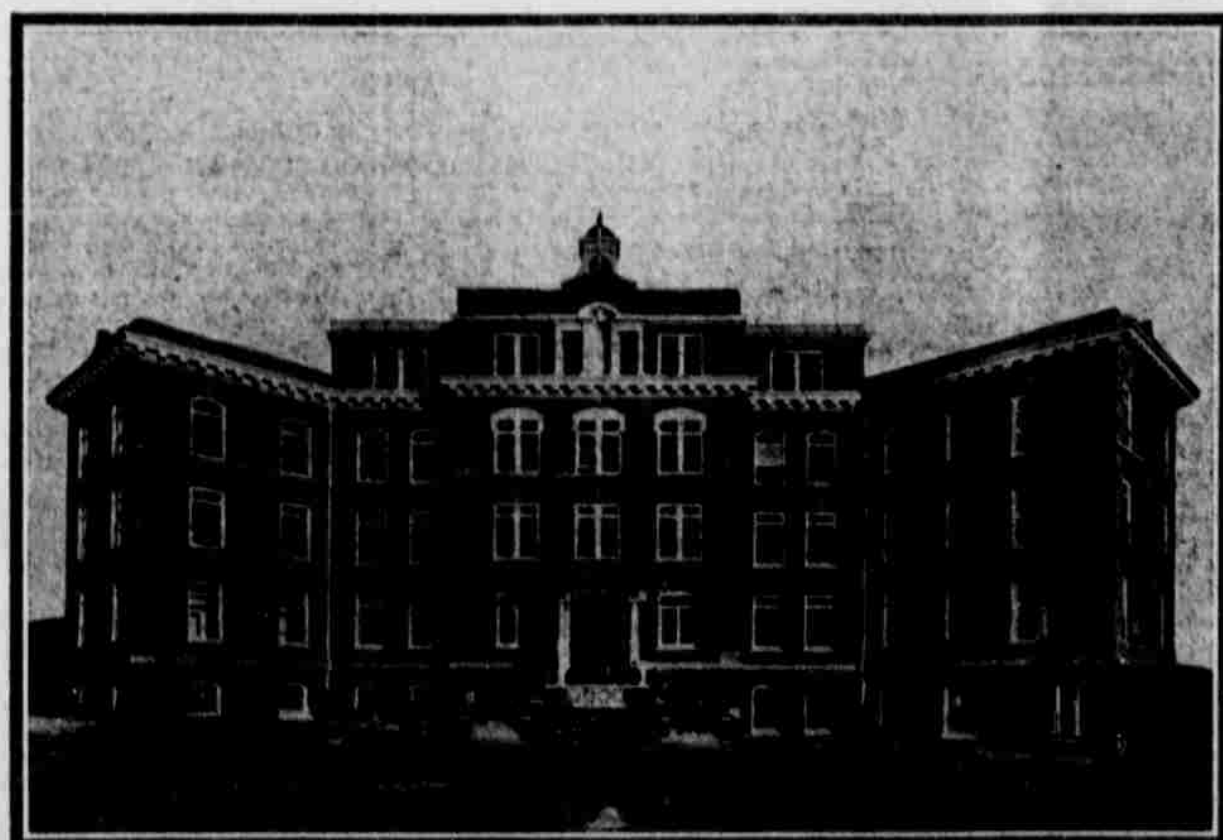
Steep grade from East Main to Sacred Heart hospital so deep with mire as to be practically impassable. It is up to the city to provide an adequate road.
