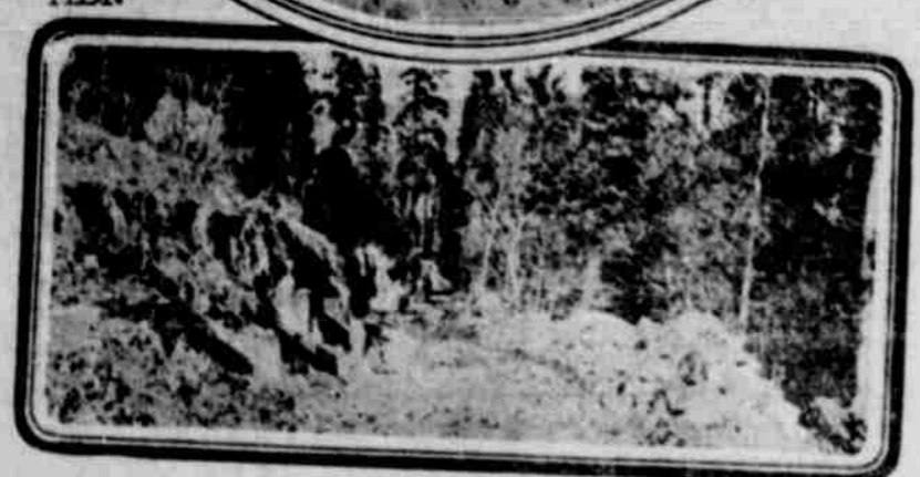
SECTION OF ROCK WORK
