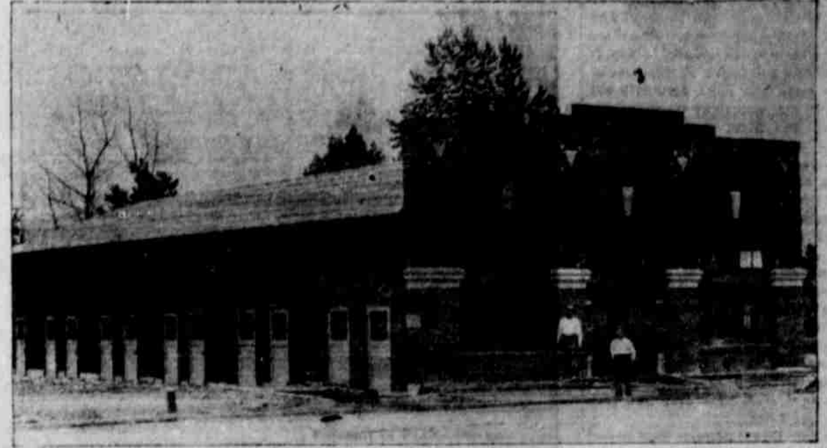
Exterior of Public Market
