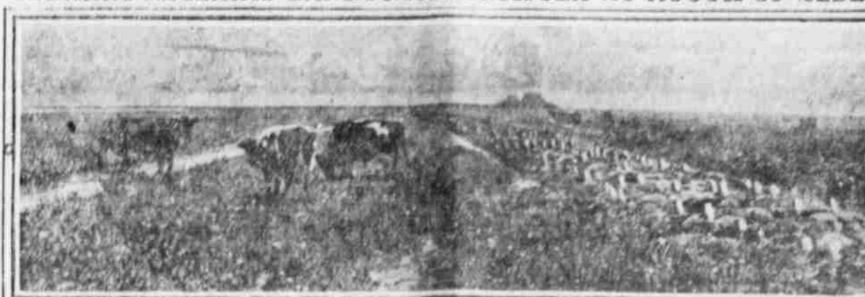
THE RESULT OF TEN YEARS' LABOR — THE SAME BREAKWATER AS IT APPEARS IN 1912.
