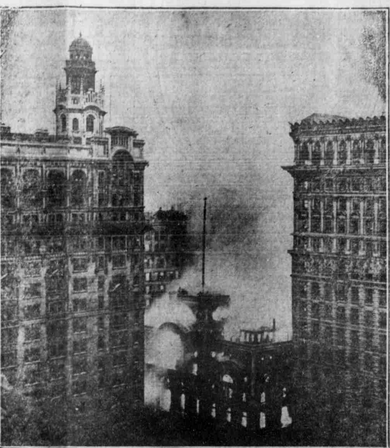
Five persons were killed and $30,000,000 damage done in the total destruction of the Equitable Life Assurance Society's building, covering an entire block in the lower part of New York City. The accompanying photograph shows the fire at its height.
