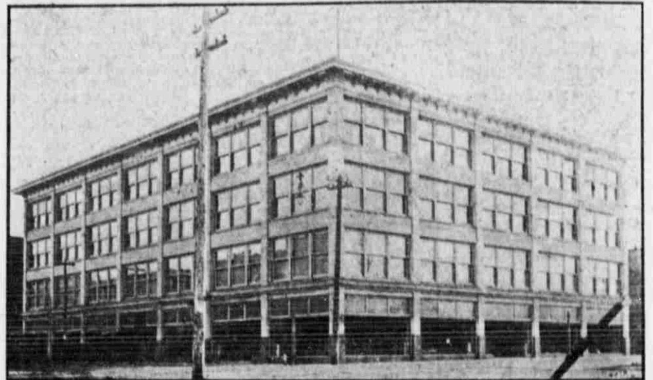
MEDFORD FURNITURE & HARDWARE BUILDING
