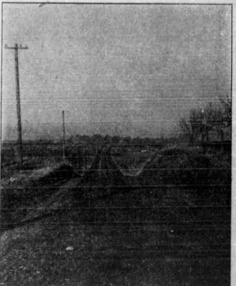
Macadam roads constructed by county, showing stages of construction.
