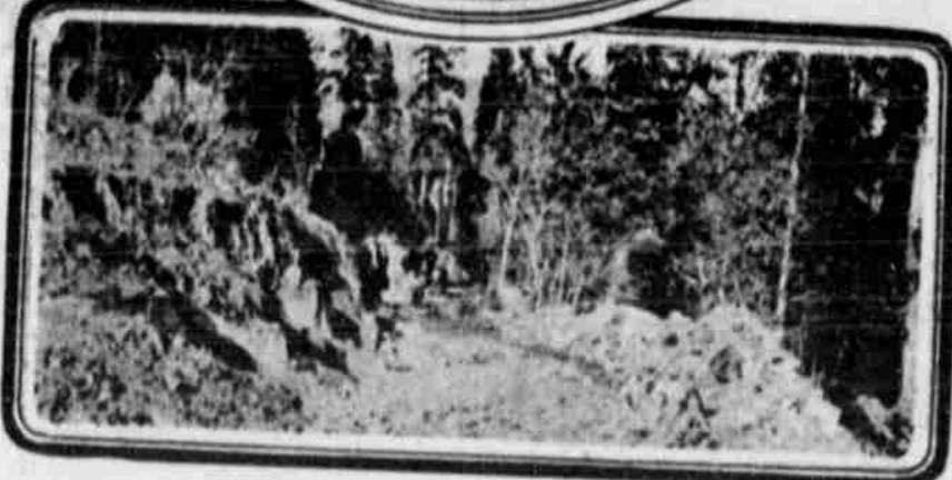
SECTION OF ROCK WORK
