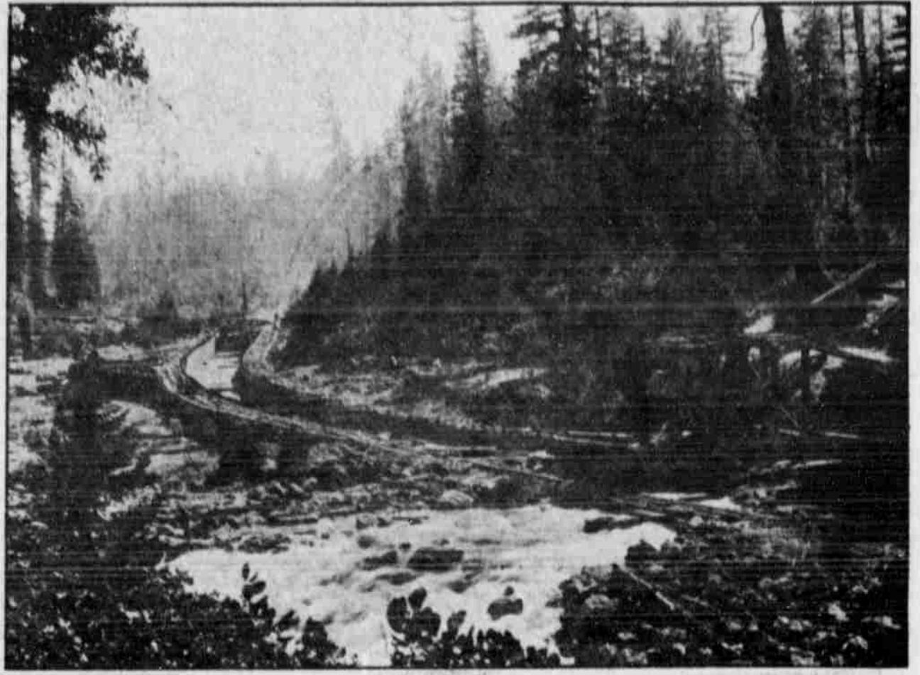
Diverting Dam, Intake Gates and Initial Section of Flume, Showing How Water Is Diverted From the Main Channel.
