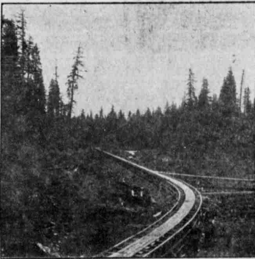
Flume Carrying Water From Diverting Dam to Power Drop.
