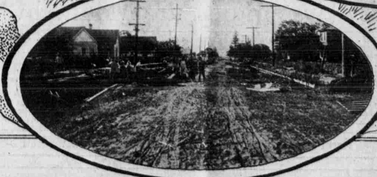
Paving Scenes in Medford, Showing the Clark & Henery Construction Stable, Paving Plant, Concrete Gang, Binder Gang, Concrete Mixer, Surfacing Gang and Curb and Gutter Crew.
