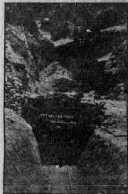
Mouth of Tunnel, Lime Kiln.
