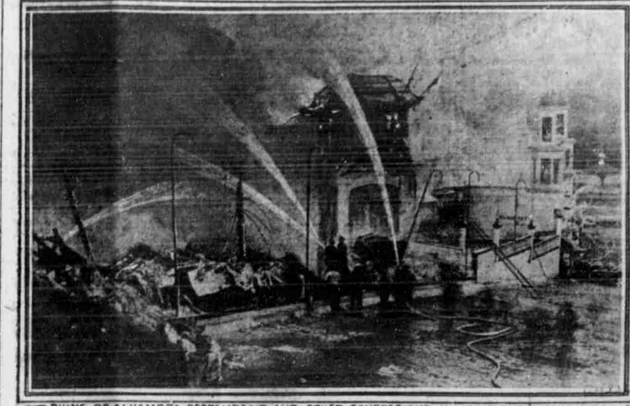
RUINS OF ALHAMBRA RESTAURANT AND OTHER CONCESSIONS IN LUNA PARK Luna park, in the heart of Coney island, was partially destroyed by fire, with a loss of $50,000. Luna park is one of the most picturesque show places on the island and several million dollars are invested in this amusement park.
