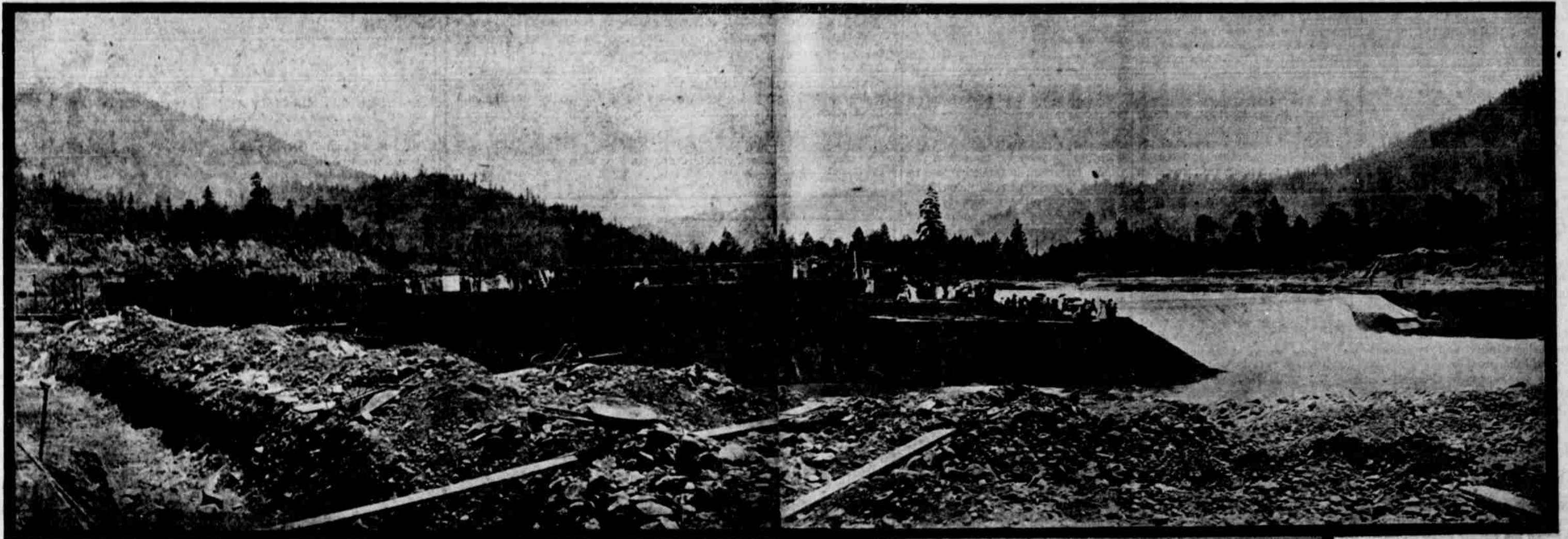
GENERAL VIEW OF THE DAM.
