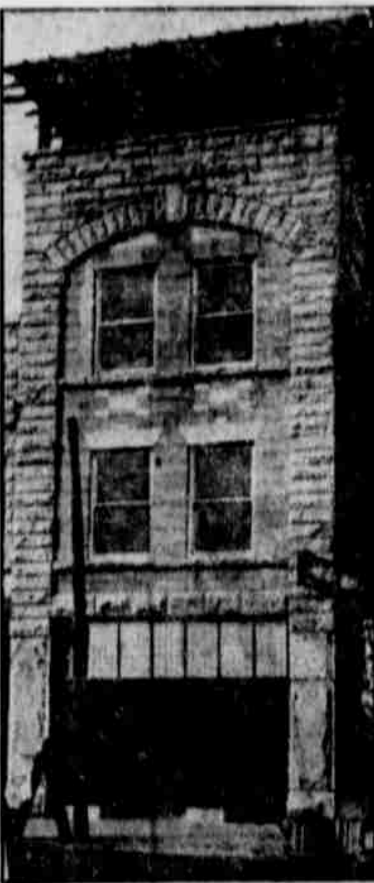
A structure built by the Rogue River Electric company of Rogue river granite.
